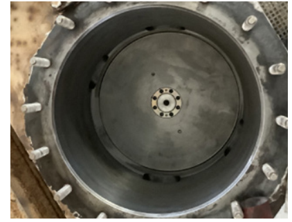
Compressor internals inspection.
