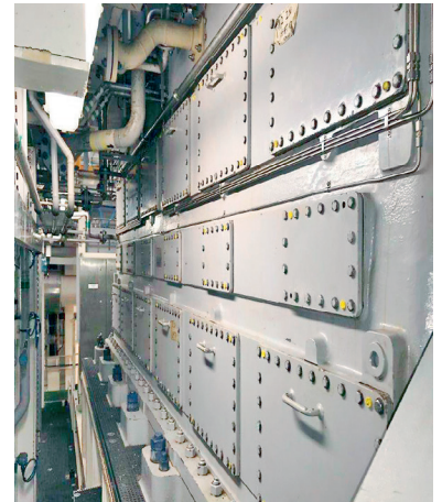
Compressor after service of just 13 days.
